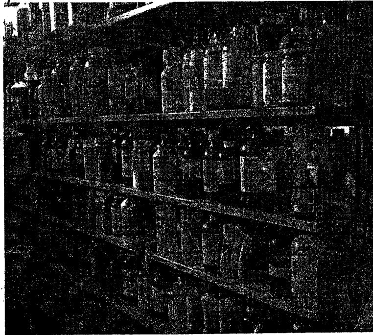
Photo 5: Alphabetically arranged lab chemicals without any seismic containment precautions.
